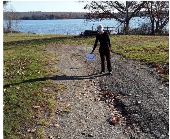
Roads and driveways built to access new development can deliver large quantities of sediment and attached P if not built correctly or maintained properly. (Photo Credit: CLA)
